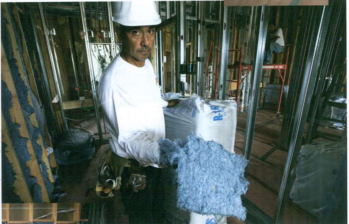
The product of recycled blue jeans: Ultratouch—a highly effective insulator
